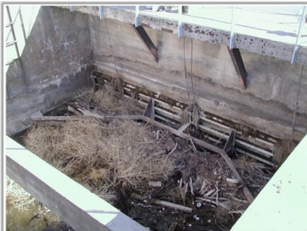
Debris and damage behind headworks' radial gate
