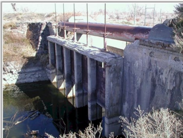
Concrete damage on out of headworks (back side of gates)
