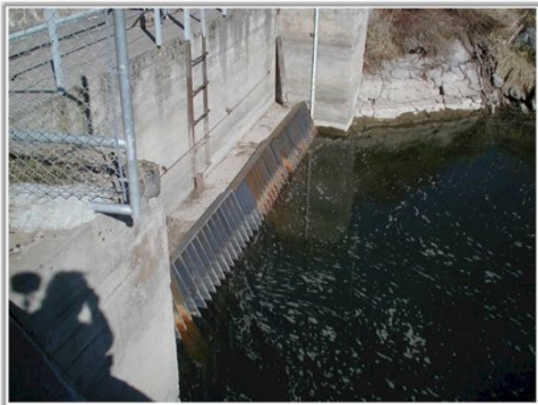
Trash rack before headworks
